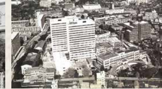
National Medical Center Hospital
