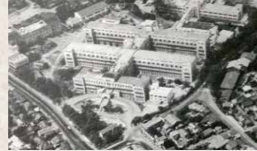
Relocated to the present site (1929)
